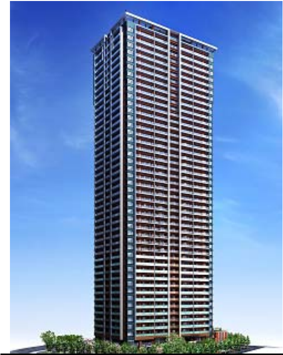
OSAKA FUKUSHIMA TOWER (Osaka-shi) Complete FY2010 Total 540 units Share30%
