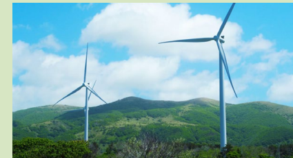
ReENE Matsumae Wind Power Plant
