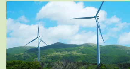
ReENE Matsumae Wind Power Plant
