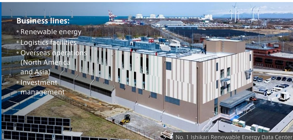
No. 1 Ishikari Renewable Energy Data Center
