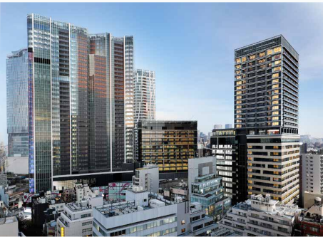
Shibuya Sakura Stage, completed in November 2023
