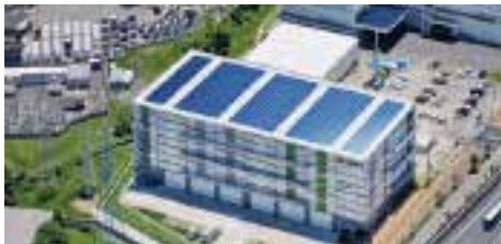
ReENE LOGI'Q Hirakata Solar Power Plant, a project involving a power purchase agreement (PPA) model that promotes demand-driven renewable energy development
