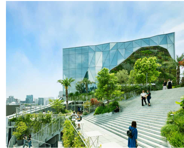
Tokyu Plaza Harajuku “Harakado,” opened in fiscal 2024. The open-air rooftop garden overlooking the Jingumae intersection is popular with visitors
