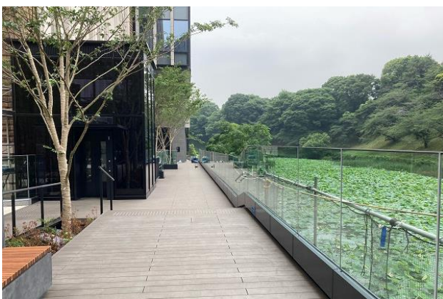
Moatside Terrace (Terrace Along the Moat)
