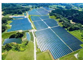
ReENE Chonan Solar Power Plant (Chonan Town, Chiba Prefecture)
