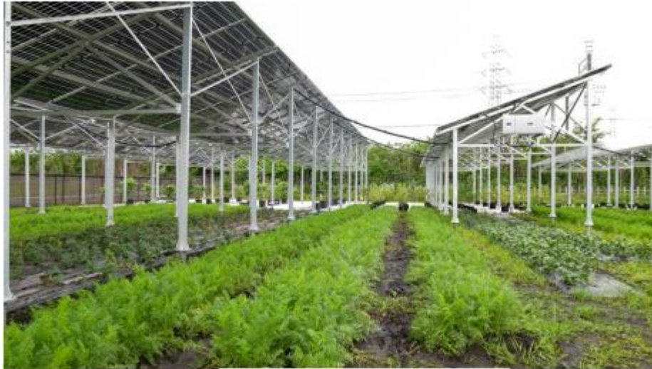
ReENE Solar Farm Higashi Matsuyama
