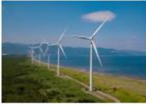
ReENE Zenibako Wind Power Station (Otaru City, Hokkaido)
