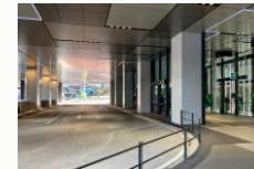
Development of a bus terminal (Shibuya Fukuras)
