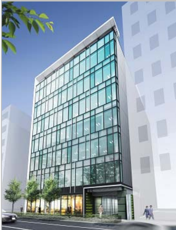
Ikebukuro Higashiguchi Project About 5,000m 2 Open FY2011
