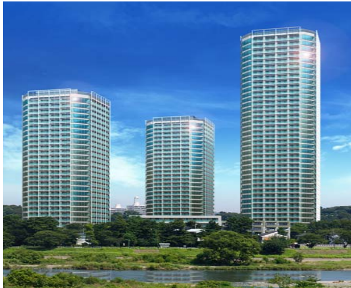
Futako Tamagawa rise Tower & Residence (Setagaya-ku) Complete FY2010 Total 1,033 units Share 30%
