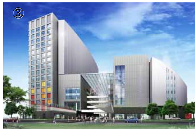
FutakoTamagawa Redevelopment About 107,000m 2 Open FY2010
