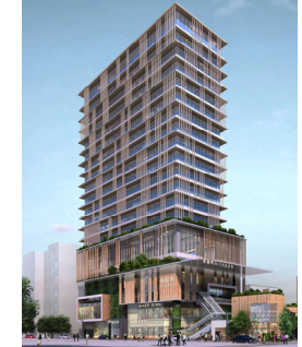
Chayamachi B-2 Block Urban Redevelopment Project Osaka Commercial, etc.
