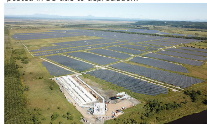
Suzuran Kushiro-cho Solar Power Plant : 92MW (Operation started in February 2020)
