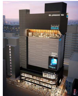
Q Plaza Ikebukuro Toshima-ku Commercial/Cinema Floor space : 17
