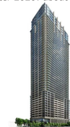
BRANZ Tower Umeda North (to be completed in January 2020)
