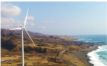
ReENE Matsumae Wind Power Plant
