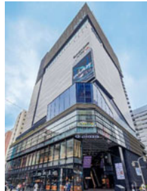
Q Plaza Ikebukuro Toshima-ku Commercial/Cinema Floor space : 17
