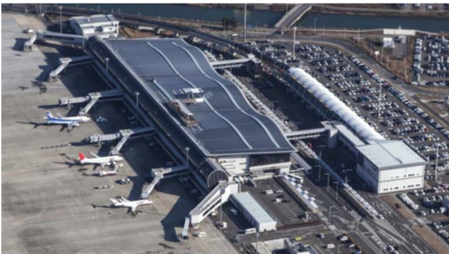
Sendai International Airport passenger terminal building Operation to be started from fiscal year 2018
