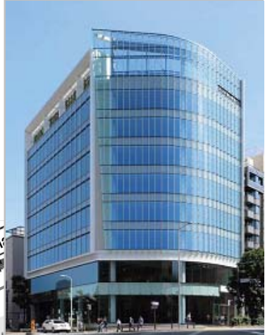
Spline Aoyama Tokyu building Opend July-2012
