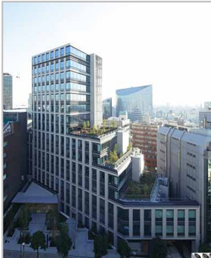
Shin-Meguro Tokyu building About 22,000m 2 Opened Dec -2012
