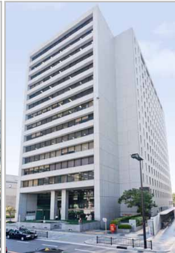
Osaka Nakanoshima Building About 34,000m 2 Acquired jointly with Activia Properties Inc. in January 2013 (equity: 50%)
