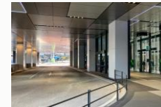
Development of a bus terminal (Shibuya Fukuras)
